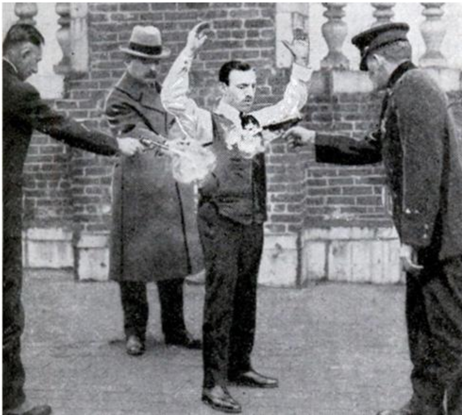
Figure 1. This photograph from circa 1897 depicts low-velocity bullets being fired into Casimir Zeglen’s torso during a test of his newly invented silk ballistic protective body armor (Oleksiak, 2020).
